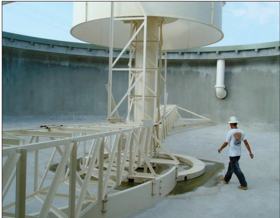
With the help of WesTech's COP™ clarifiers, Pace Water System was able to increase capacity, simplify operations and provide for effective nutrient removal.
