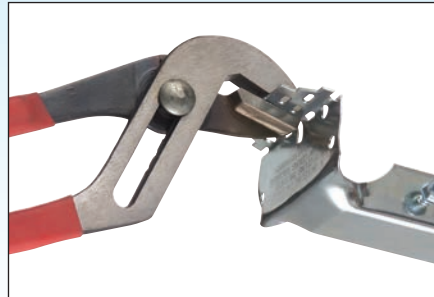
Bracket ends are pre-set for a 1/2" ceiling. For other ceiling depths, bend the bracket ends along the appropriate score line.
