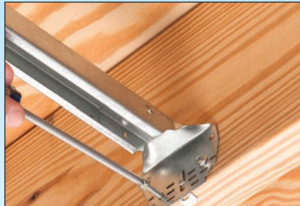
Bracket mounts securely to joists.
