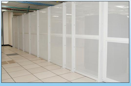
Custom Data center Privacy System based on customer requests; features a steel frame with rigid mesh
