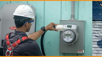
1 A PV-ready socket installed at the electrical meter makes system interconnection safe and easy.
