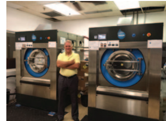
Julian Ramirez, Owner of Inverrary Resorts, Fort Lauderdale, Florida has installed 2 Xeros washing machines and 1 Xeros branded dryer at this location.
