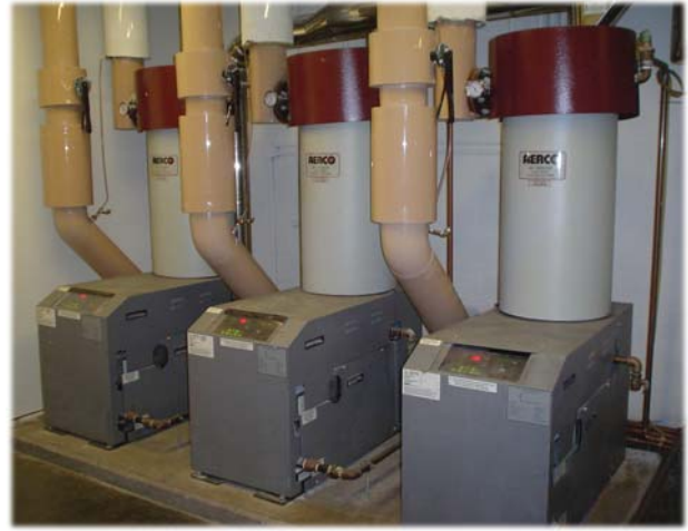
AERCO KC1000 boilers & water heaters now have a 20:1 turndown ratio for heating loads from 50 MBH up to 1000 MBH
