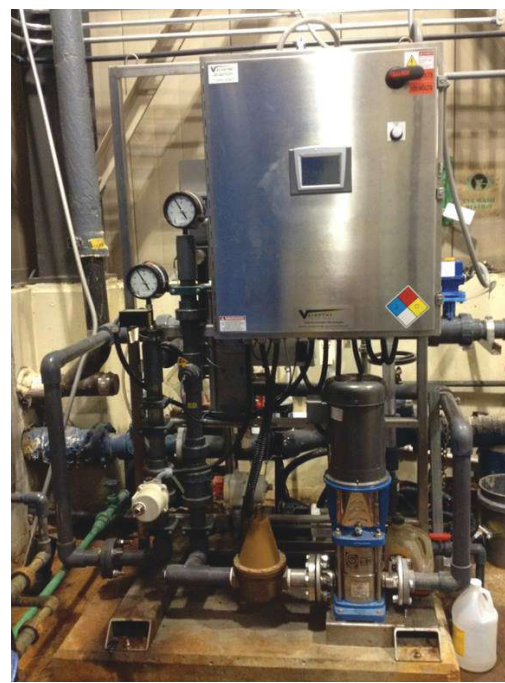
At the Westerly plant, a polymer blend unit makes a polymer solution for the CEHRT process.
