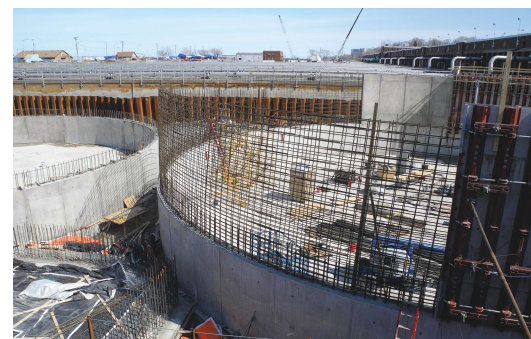
Construction at the Easterly Wastewater Treatment Plant (March 2015) to expand secondary treatment capacity as part of the Project Clean Lake consent decree with U.S. EPA.
