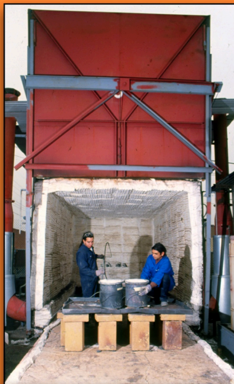
Multiple furnaces for parts up to 8 feet wide and 25 feet long
