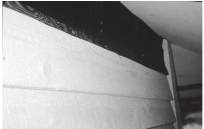
Figure 220. This figure indicates a sequential step from figure 218. The battens have been carried up to the soffit. As the finished siding approaches the top of the wall a single or double vent can be used. The choice is only determined by the desired "look" and/or performance. Only experience will tell how much ventilation is necessary or appropriate. Cut a strip of fiberglass insect screen to be stapled to the top leading edge for the last "common" siding course above the reveal line of the existing course of siding. This sequence is then followed by using cutoffs of the furring material. Use \frac{1}{2} inch pressure treated plywood, ripped to a width of 2\frac{7}{8} inches. A wide strip is used to increase the width of the nailing base. Keep the nails at least 1 inch away from any end of a board to decrease the likelihood of splitting the siding.
