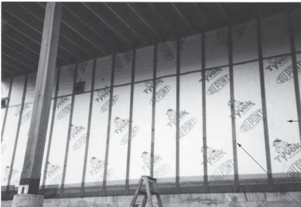
Figure 218. A framed example of backing side of exterior ventilated cladding.
