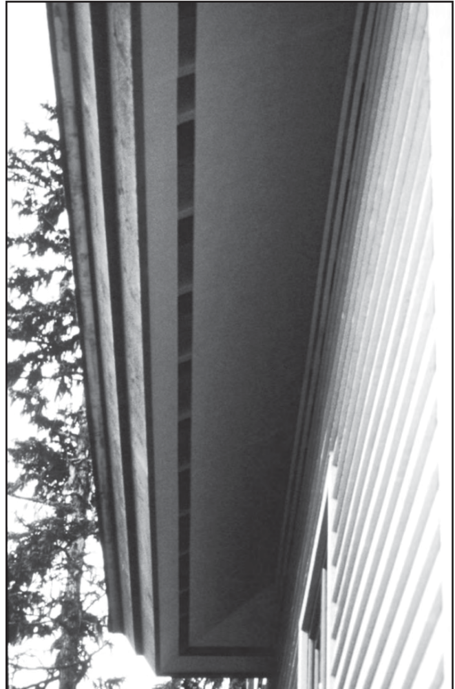
Figure 221. The stand-off furring blocks are attached over the sandwiched screen and original furring. The corner boards have only the original furring underneath them. This gives a nailing base for the corner board and the siding that will butt into the corner board. As the stand-off blocks at the top of the wall are installed, do not install a furring block where the siding is going to marry to the corner board, as this will result in the siding standing out proud of the corner board. The siding is formed, faired, and bent from the corner board plane to the next stud-furring spacer so the air space goes from nothing to the 1/2 inch space depending on the stud spacing. This holds true when a deck or other mid-wall penetration occurs. Visually it is quite undetectable.
