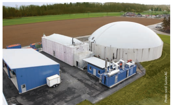
Biogas plant in Switzerland.
