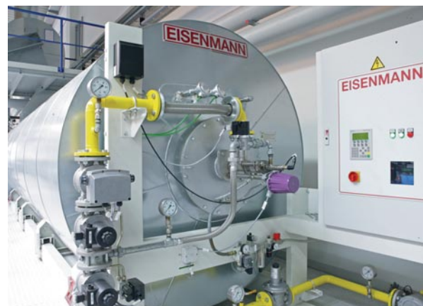
Thermal incinerator for exhaust air purification
