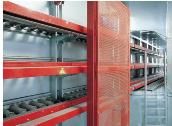
Fig. 4: Roller drive (center) and bearing are located outside the furnace
