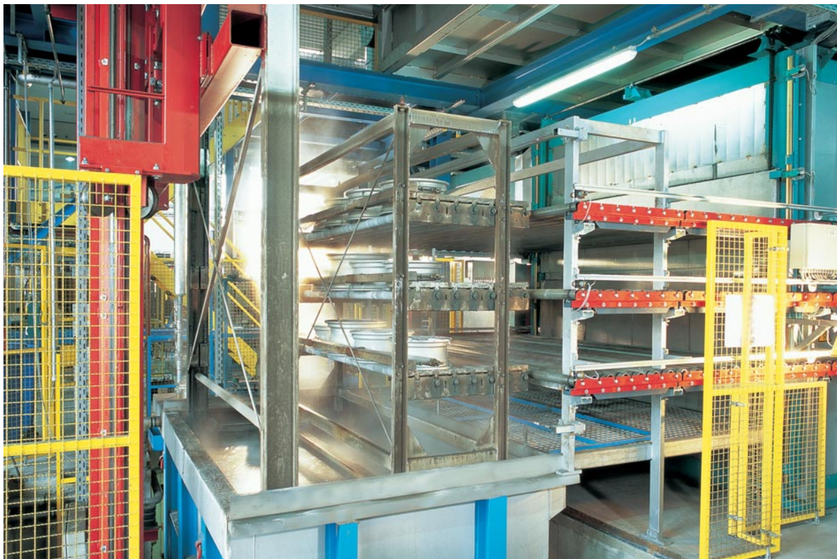
Fig. 5: The quenching basin is located directly underneath the annealing furnaces
