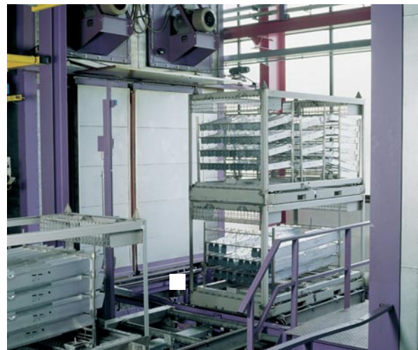
Fig. 10: Aluminum sections are transported through this ageing furnace in a wet chemical treatment line in baskets stacked two high
