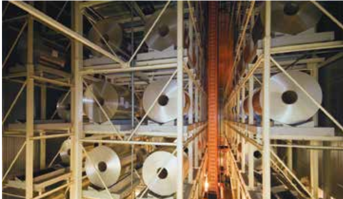
Aluminium coil store holds over 400 coils of premium grade aluminium at any one time
