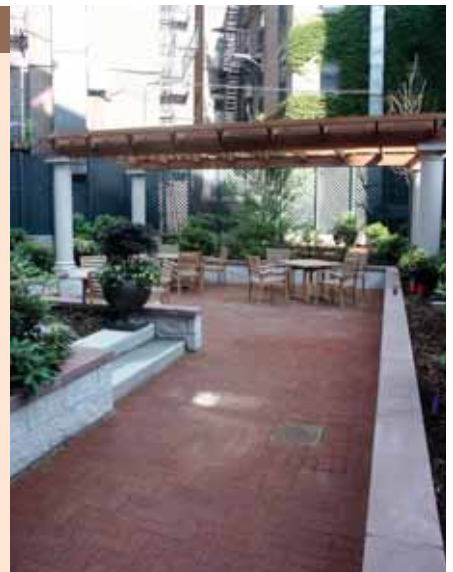
An urban landscape shines with a brick patio and segmented retaining walls capped in pigmented concrete. This traditional arbor, constructed of cedar with cellular PVC posts, blends beautifully with the dark green lattice installed for screening.
