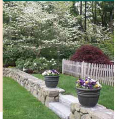
A natural fieldstone wall with granite steps creates a terrace on a flat grade. The picket fence adds a rustic touch to this well-organized hardscape.
