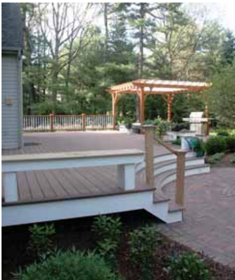
An aged brick patio gets a modern boost by the addition of a large, composite deck with white trim. The pergola, constructed of cedar, gets a two-tone finish to match.
