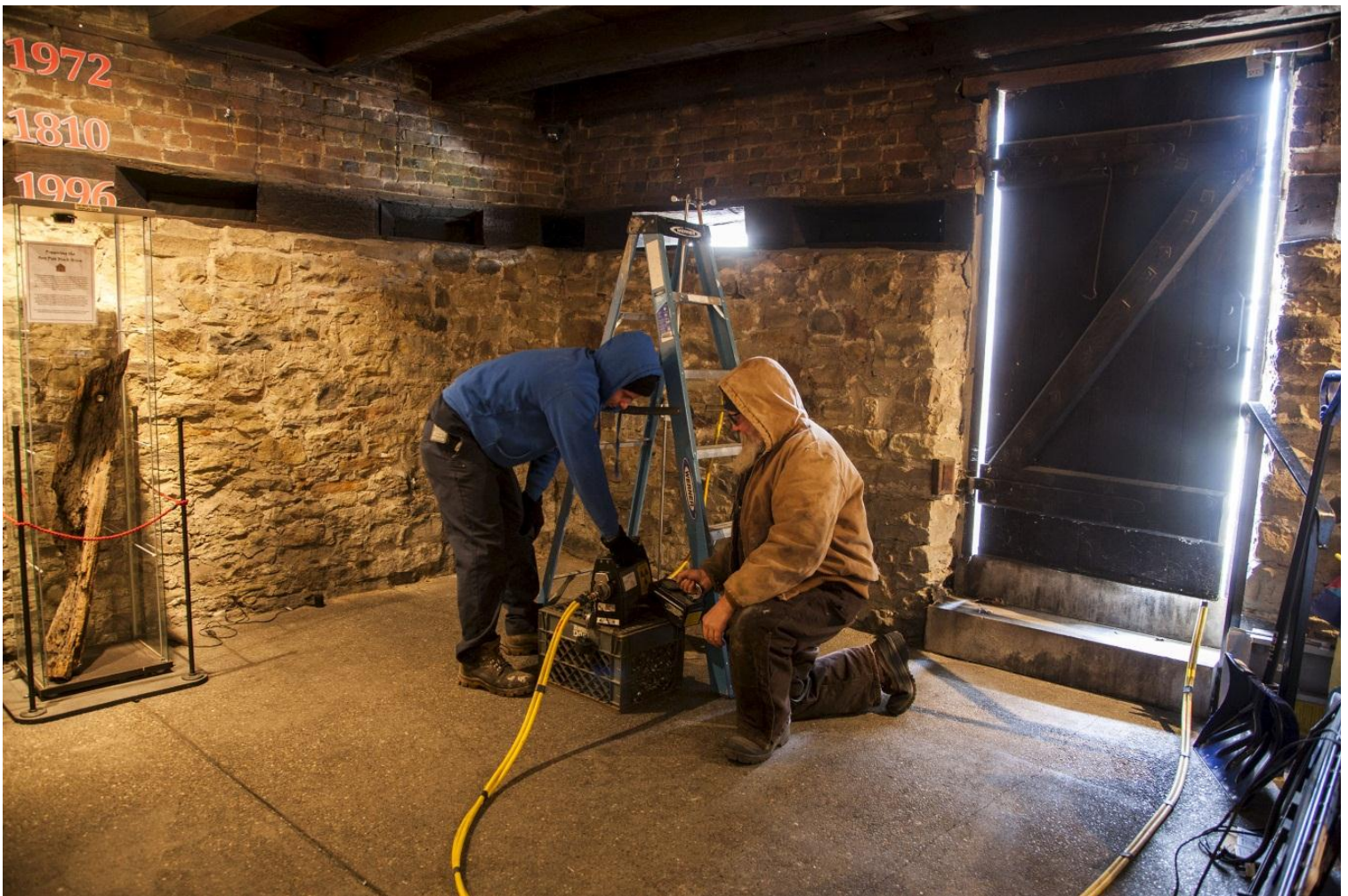
Radiographic crew members Jake Fetchin, Assistant Radiographer, (left) and Phil Martin, Radiographer, (right) are performing a radiation survey of the equipment to ensure the radioactive material is returned to its safe and shielded position.
