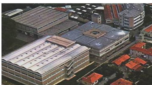
Figure 1 Gentium S.p.A. MANUFACTURING FACILITY
