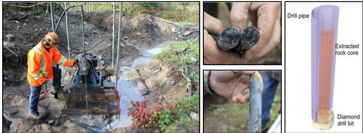
Figure 23 TRIO'S EXPLORATORY DIAMOND DRILLING
