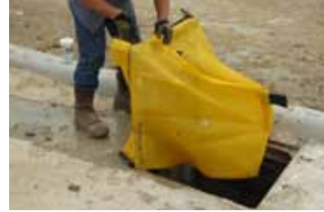
Slide Siltsack® over opposite side of grate.
