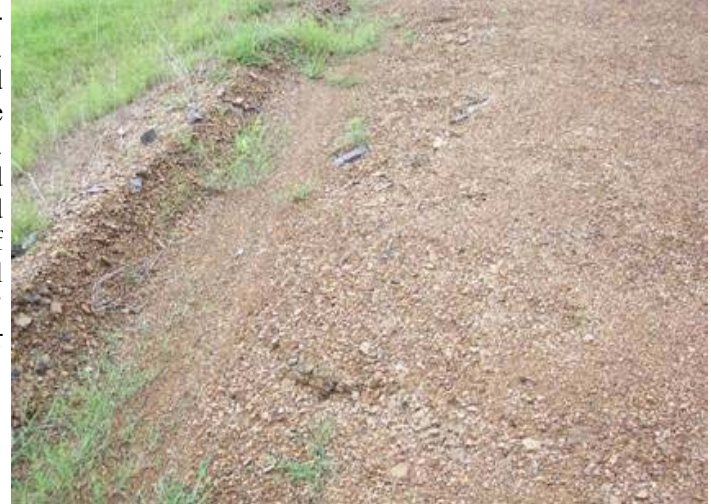
Little or no visible erosion after 740 Silt Stop powder application
