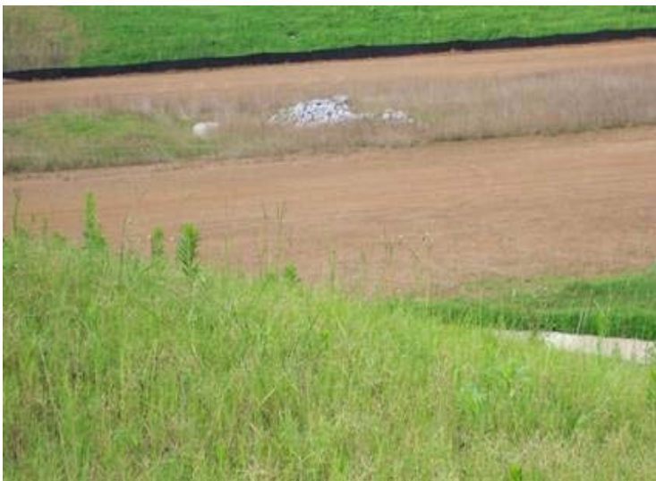
Disturbed road bed treated with APS 740 Silt Stop powder
