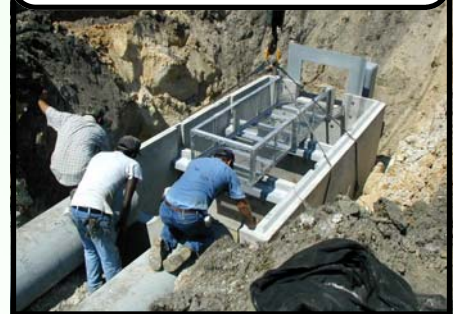
Step 2: Hook up pipes
