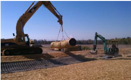
Flexamat roll being lifted
