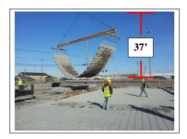
PaveDrain Mats were 7.5' x 32.2' and weighed 11,500 lbs. The Spreader bar weighed an additional 3,500 lbs.
