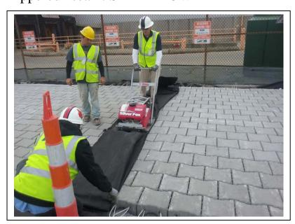
Step #7 The PaveDrain Mats can be "tailored" to accommodate a variety of different obstacles within the "working area". Each site is different but some examples of obstacles can be: water meter openings, man-holes, existing curb drains, light posts, sign posts and/or existing concrete structures. The specified PaveDrain mats can be "tailored" by removing individual units within the mat (before the mat is installed *OR* after the mat is installed). SEE EXAMPLES BELOW.
