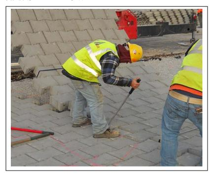
Step #5 If Submittal pack requires the use of PaveDrain "Lock Block" and/or "Lock Block Rows" you will need a 4 ½" dia. angle grinder (w/ masonry blade). SEE PHOTOS BELOW & OPTIONS ON DETAIL PAGES AT END OF PACKETT.
