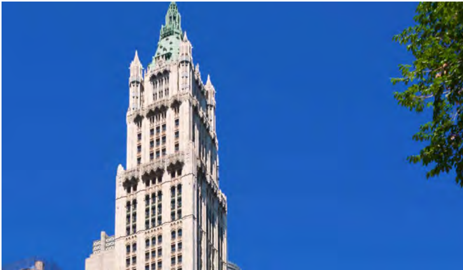
Loan number 12, the Woolworth Building, is expected to refinance despite several leases coming due.
