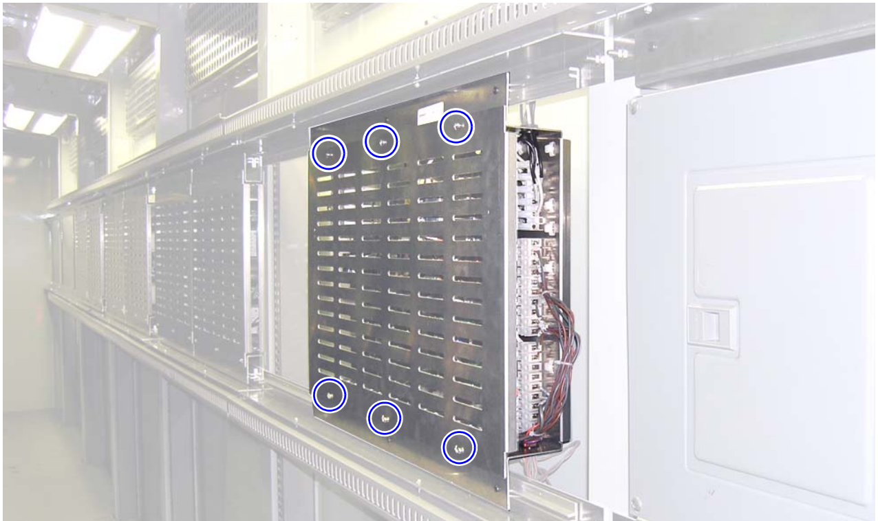
Figure 9. Screw locations on the controller’s cover.
