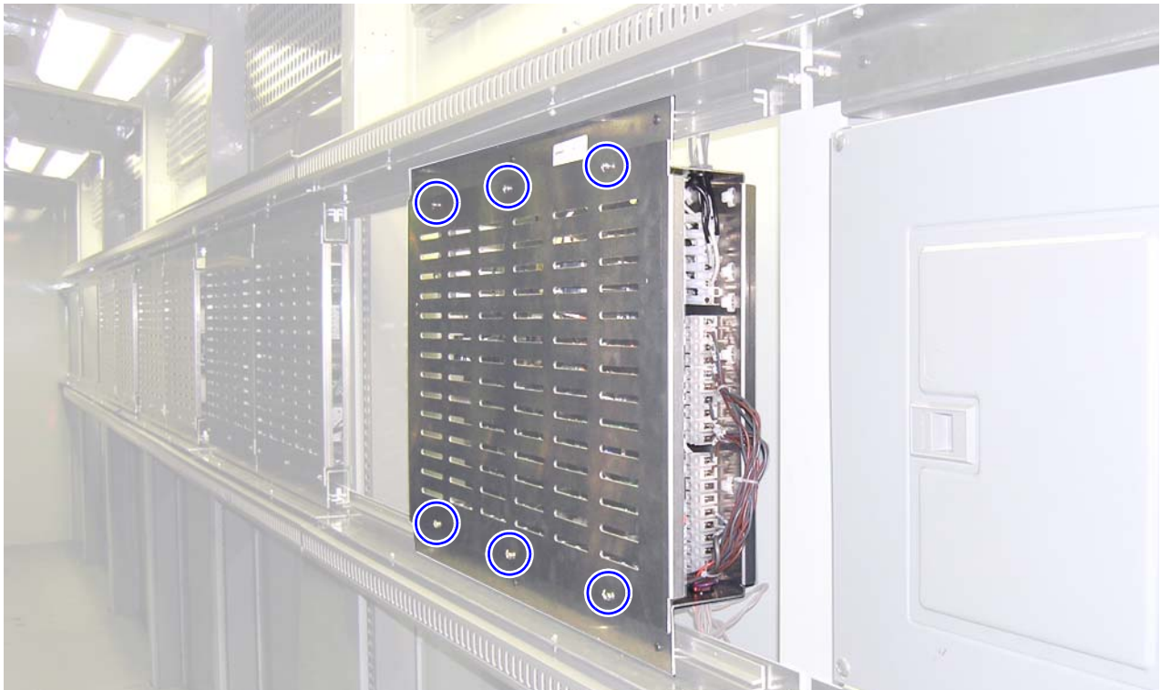
Figure 21. Locations of the screws on the controller plate's cover.
