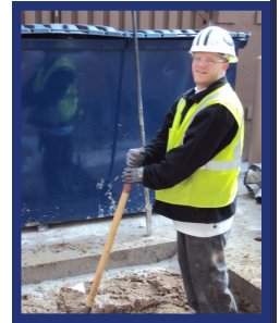
Mike Fernandez digging trenches at Children's Hospital in February
