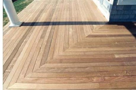
A wood stabilizer has been applied to these boards to minimize minor surface checking. This area will be left to weather naturally.
