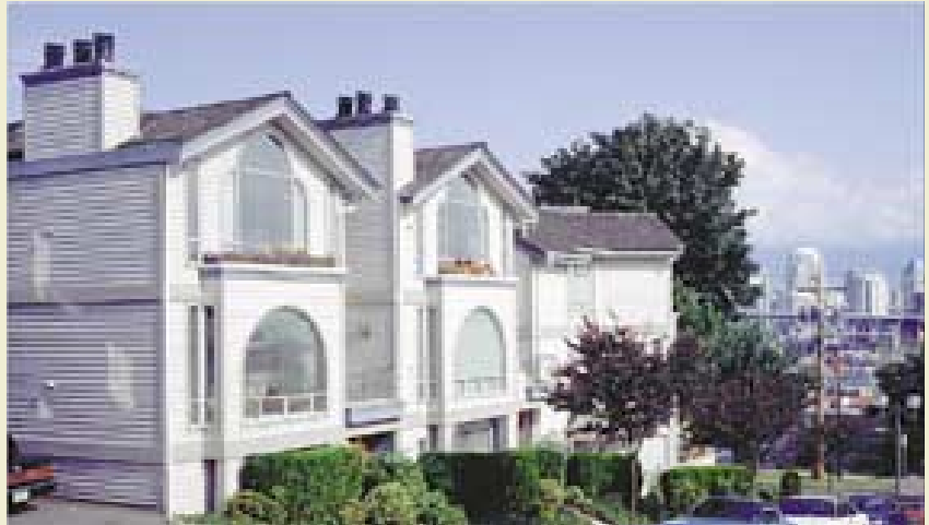
PHOTO 4: The Windgate townhouses near Choklit park in Vancouver, BC use decorative exterior fascia boards at the floor level, combined with sloping roofs and overhangs as part of a moisture management strategy.
