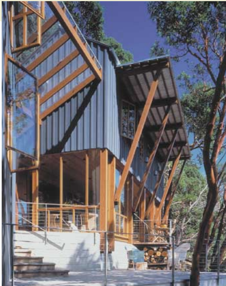
PHOTO 3: Girvin Cabin – This wood-frame studio and house located on Decatur Island, Washington uses pronounced overhangs that are both functional by deflecting rainwater from a window wall and architectural to suit the surrounding environment.
