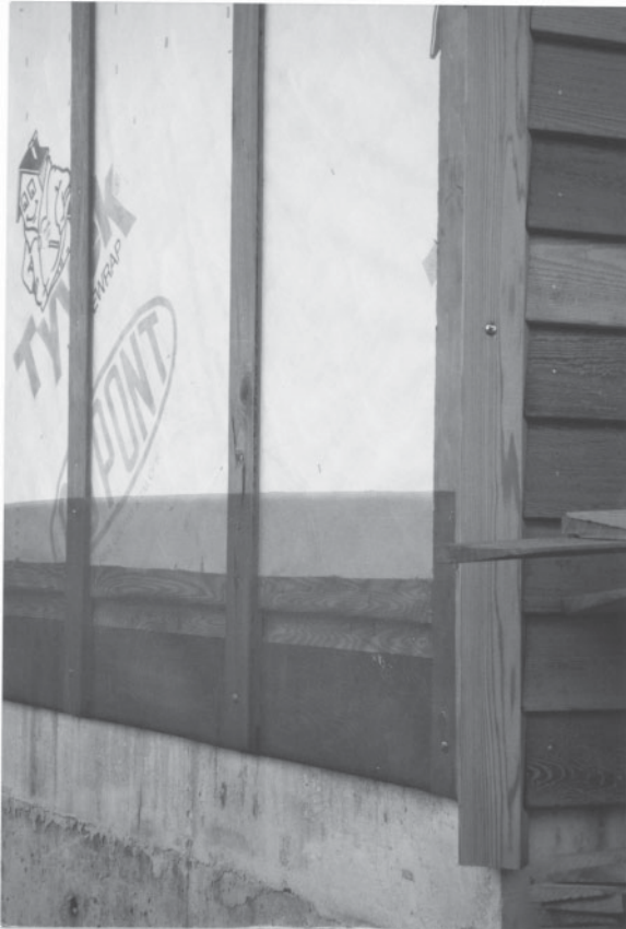
Figure 219. Shows the installation of insect-proof mesh vent screening installed over the bottom opening of the ventilated wall. This allows air and water drainage to easily occur behind the exterior rain-shield sheathing.
