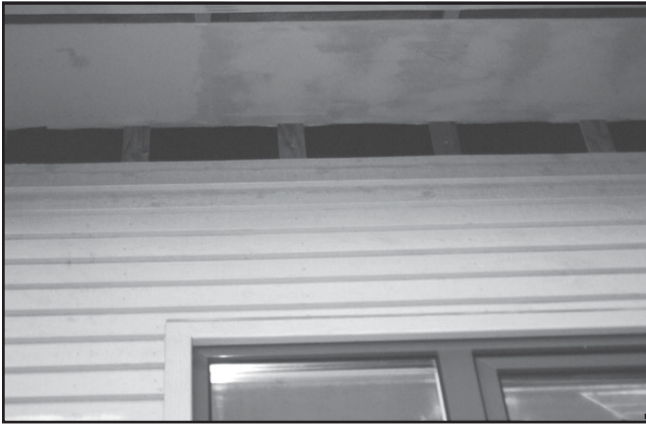
Figure 221. The stand-off furring blocks are attached over the sandwiched screen and original furring. The corner boards have only the original furring underneath them. This gives a nailing base for the corner board and the siding that will butt into the corner board. As the stand-off blocks at the top of the wall are installed, do not install a furring block where the siding is going to marry to the corner board, as this will result in the siding standing out proud of the corner board. The siding is formed, faired, and bent from the corner board plane to the next stud-furring spacer so the air space goes from nothing to the 1/2 inch space depending on the stud spacing. This holds true when a deck or other mid-wall penetration occurs. Visually it is quite undetectable.
