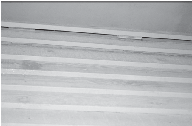
Figure 222. This is similar to figure 221. The top-most spacer is cut to not lay on the siding, but over the existing furring and insect screen. One stand-off is probably more than adequate.
