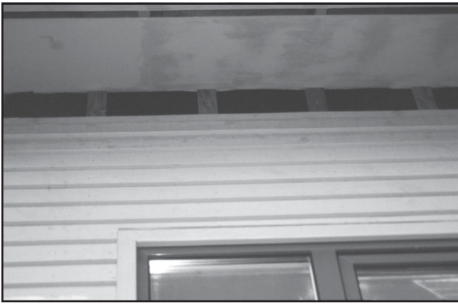
Figure 221. The stand-off furring blocks are attached over the sandwiched screen and original furring. The corner boards have only the original furring underneath them. This gives a nailing base for the corner board and the siding that will butt into the corner board. As the stand-off blocks at the top of the wall are installed, do not install a furring block where the siding is going to marry to the corner board, as this will result in the siding standing out proud of the corner board. The siding is formed, faired, and bent from the corner board plane to the next stud-furring spacer so the air space goes from nothing to the ½ inch space depending on the stud spacing. This holds true when a deck or other mid-wall penetration occurs. Visually it is quite undetectable.
