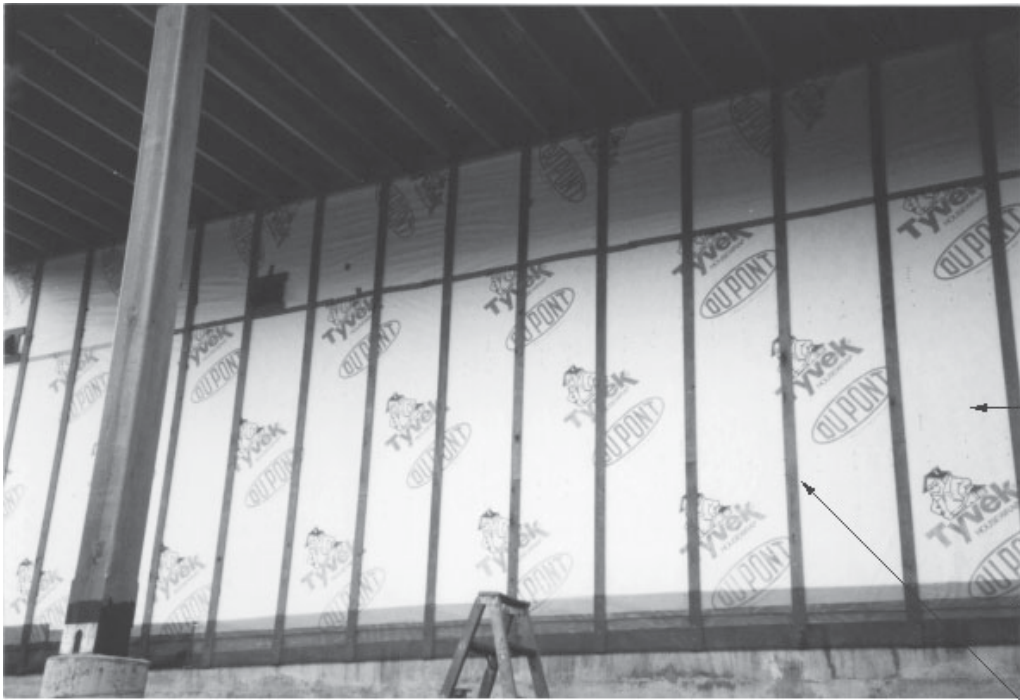
Figure 218. A framed example of backing side of exterior ventilated cladding.
