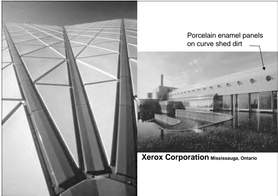
Calgary Oval Olympic Arena Roof
