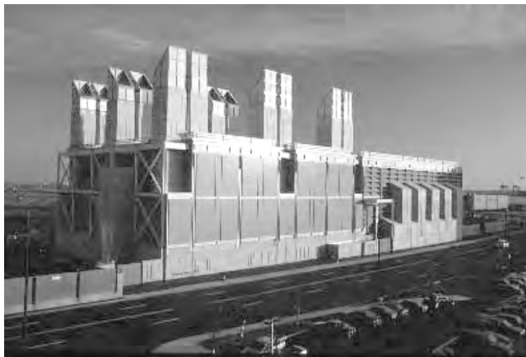
Ventilation Building No.7 TAMS/Wallace Floyd Design Group / Stull & Lee
