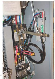
non-magnetic core, giving them perfect linearity and improved accuracy over wide current ranges, saving time on installation. The air core of Rogowski coil's eliminates the negative effect of magnetic fields which pose a serious issue to conventional CT's in similar environments.
