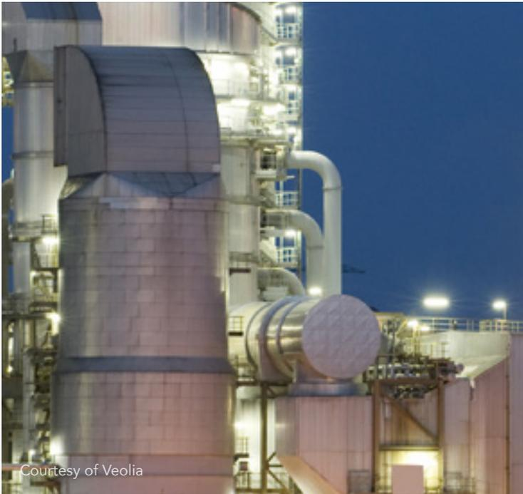
Just as electricity is distributed over networks of wires to many buildings, it is also possible to distribute heating and cooling via networks of pipes. District energy systems produce steam, hot water, and/or chilled water at central plants and, through a network of insulated pipes (often underground), distribute the steam or water to multiple buildings. District energy plants often include power generation, typically CHP, which further increases overall efficiency.
