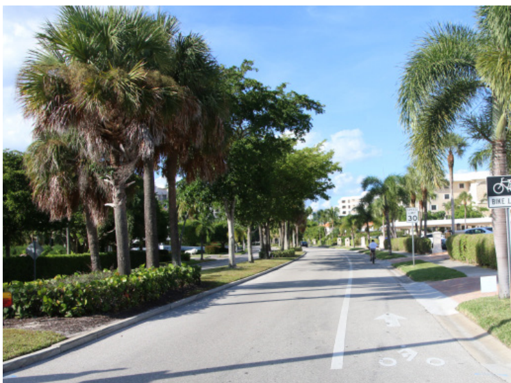
This section of Gulf Shore Boulevard (above) has overly-wide travel lanes. The travel lanes are 13 feet; the recommended travel lane width is 10 feet. Using paint the lane can be narrowed by adding a painted buffer to the bike lane.
