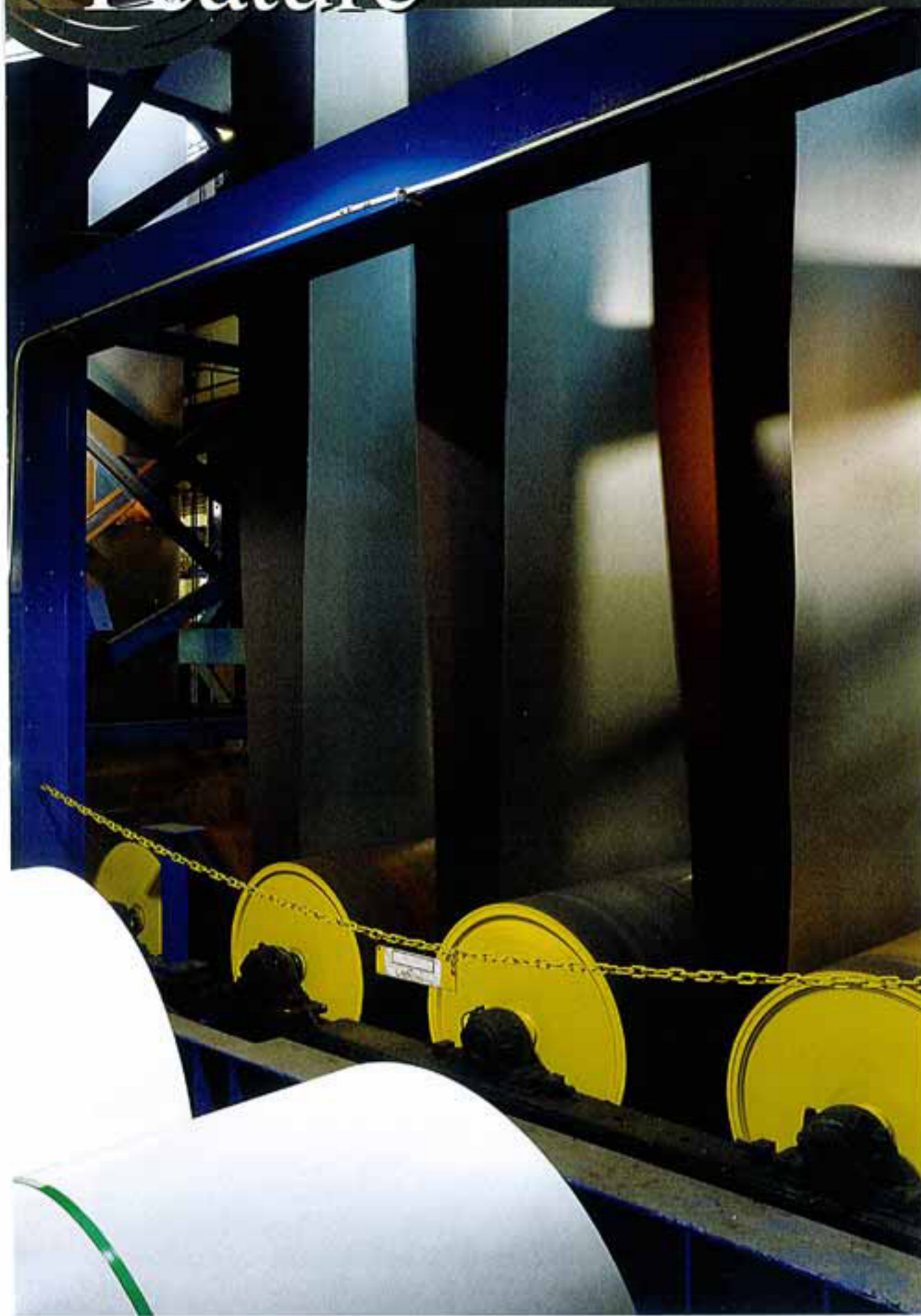
As part of Centria's Ambridge facility retrofit project was the upgrade of its accumulator tower.
