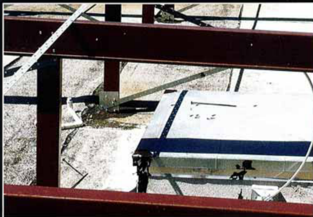
Initial steps for a Galvalume metal roof conversion of a flat roof. p. 14
