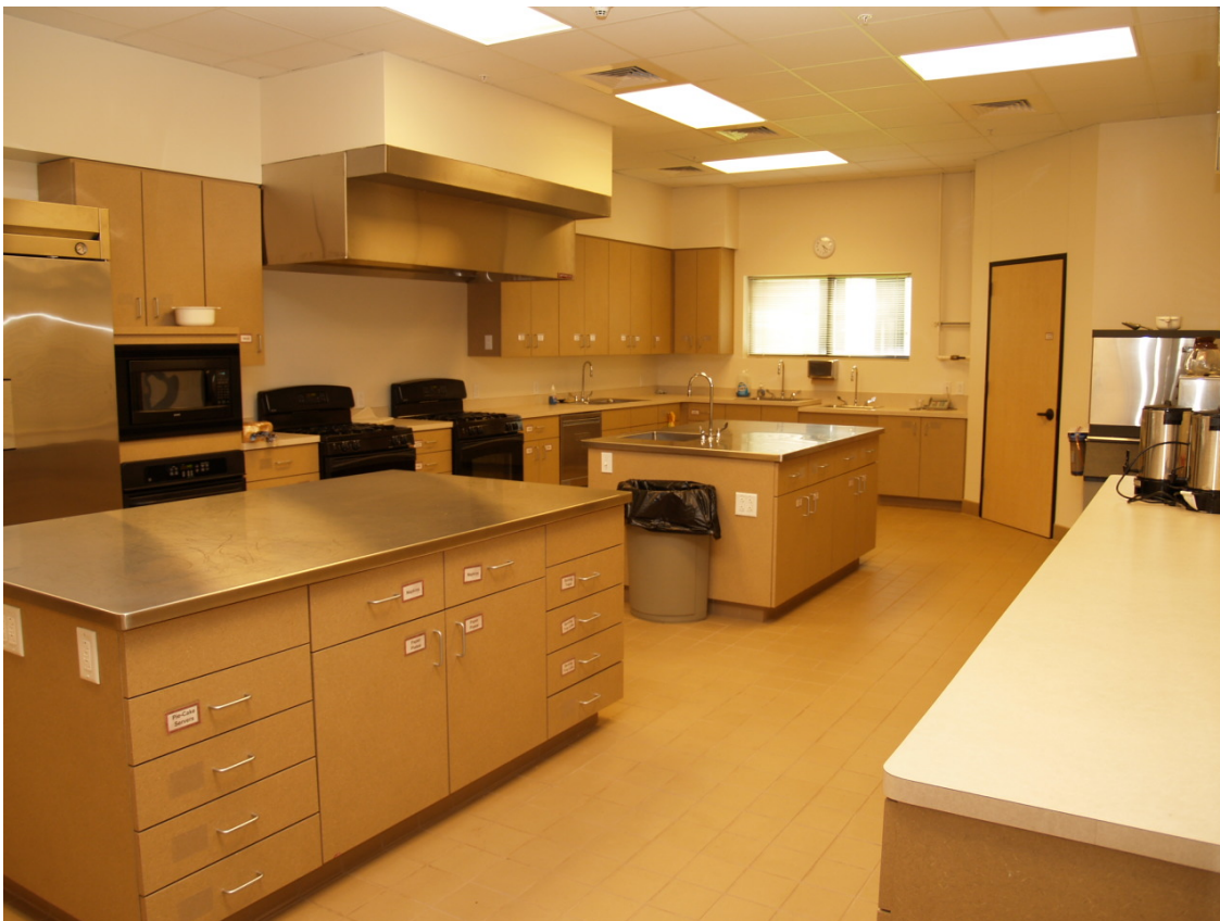
Residential Ranges with Type 1 Hood. Hood sized to later allow a commercial range.
