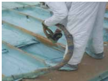
Fig. 12: Applying Closed-cell foam at rafters Fig. 13: 8.5” of foam in 2 x 10 rafters
