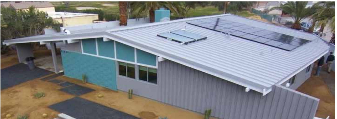
Figs. 18, 19: Completed ReVISION House™ Las Vegas
