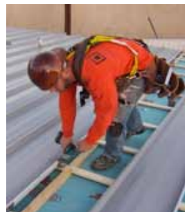
Fig. 14: Metal roof installation
