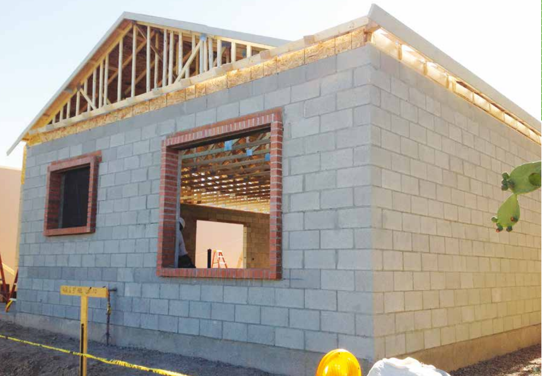
Smart Details. Bricks surrounding the window cantilever from the wall to allow space for the exterior foam insulation and three-coat stucco finish. Trussed rafters include plenty of room for mechanicals, and recycled steel framing has extremely good durability.
