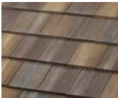
The roof of the ReVISION house is MonierLifetile's Buckskin CT Slate 900 series, a "cool roof," which means it has high solar reflectance and thermal emittance. For more cool roof options, visit: www.mlt.boralna.com
