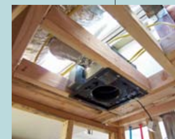
The fan in the laundry closet will be set to run constantly at a very low speed, assuring proper air changes in the urethane insulated "thermos bottle" of a house.
