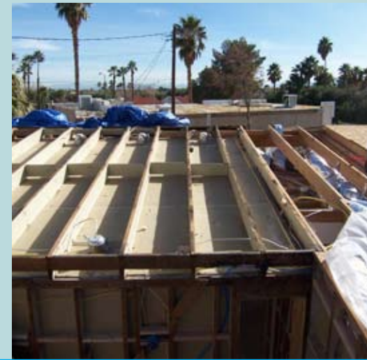
Stripped from the outside, the rafter bays over a vaulted ceiling area are ready for BASF Comfort Foam closed-cell spray insulation (below). Working from the outside makes for an unobtrusive retrofit that could be of significant value in an occupied home.
