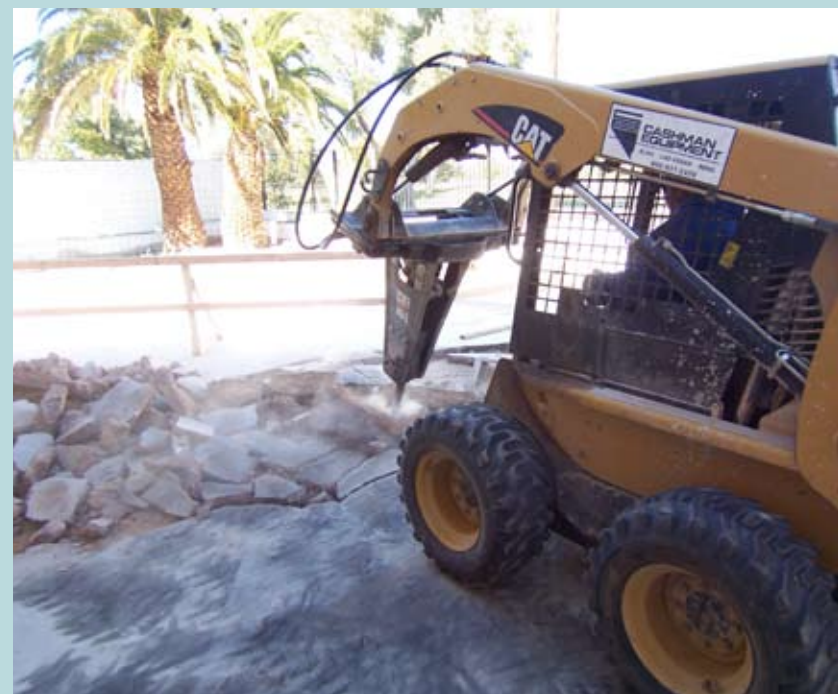
Nevada Concrete Services breaks up the existing driveway and patio at the ReVISION House (below). This concrete debris was hauled by Valley Recycling to a plant where it was ground and recycled for use in road beds.
