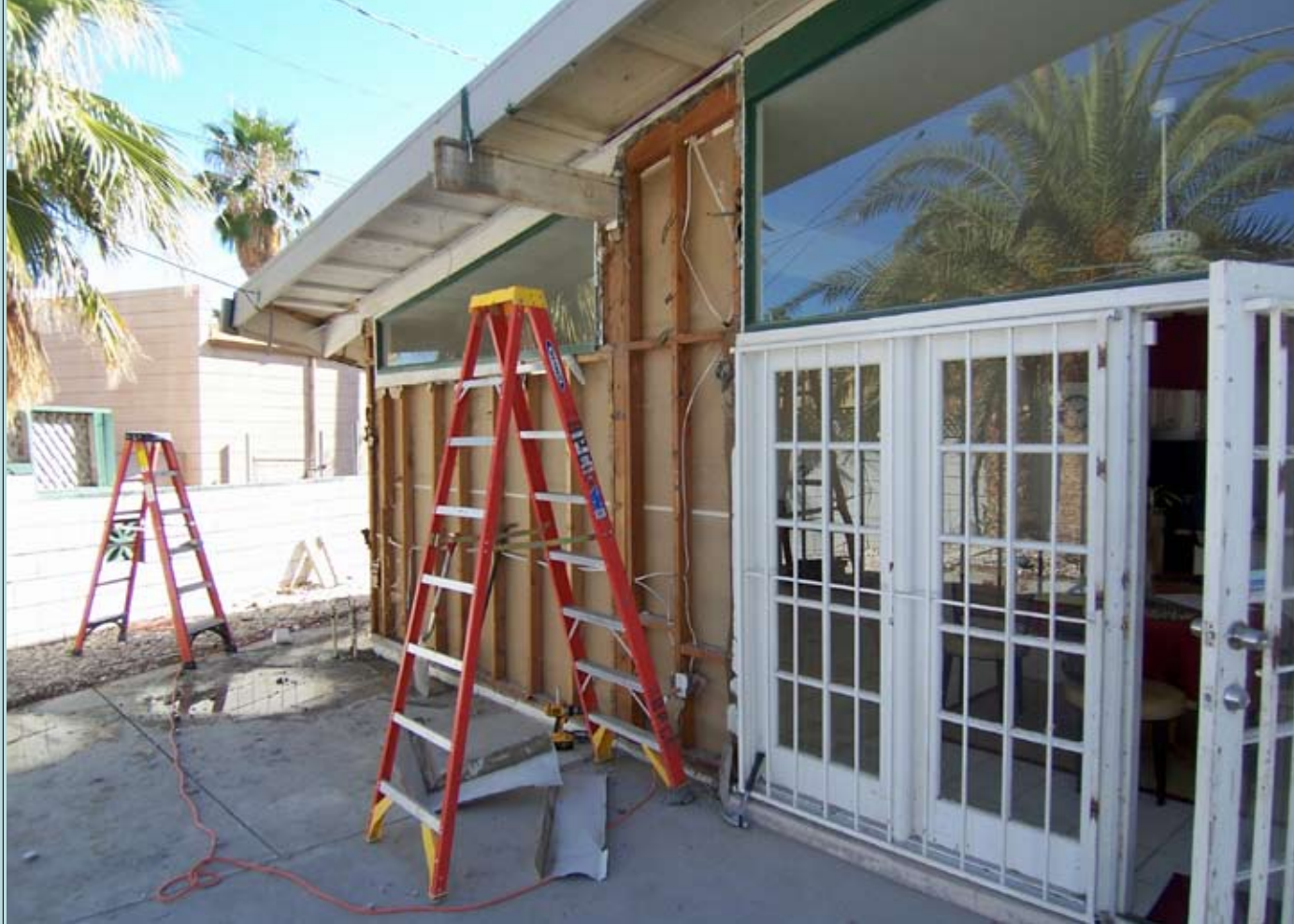
To install the holddowns for the Simpson StrongWalls, the slab edge had to be cut away (right) and reformed with an array of anchors.
