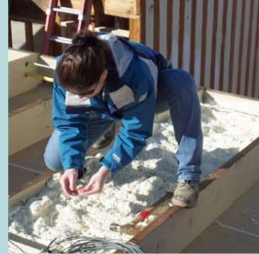
Lois Arena, an engineer from DOE's Building America team, Steven Winter Associates (above), attaches heat sensors to one of two test rafter bays. One test patch will have DuPont RoofLiner; the second will have an additional foil radiant membrane. The result will determine if it is cost effective to add the radiant membrane to the roof, which is already super insulated and capped with a low-emitting metal cool roof.
