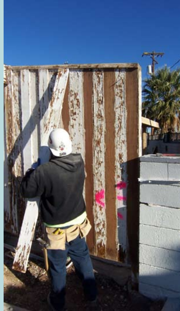
Clear redwood "batts" being carefully removed from redwood T-111 plywood (above). The Dryvit synthetic stucco system was applied with an additional layer of 1x6 foam to maintain the board and batt look, one of the design signatures of the exterior
