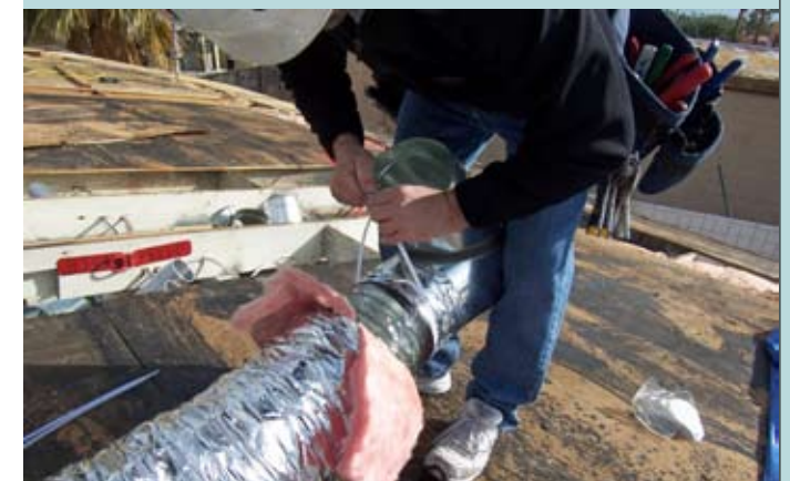
Ritchie Bedor, owner of A-Bear Air Conditioning and Heating, focuses his attention on sealing a Y-joint in the new ductwork before installing it in the conditioned attic space.
