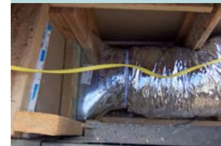
The right way to do a boot connection: Sealing flex duct to a boot requires UL-181 foil duct tape (not the usual cloth duct tape, which has a rubber-based adhesive that will dry out and eventually lose its bond). The foil tape gets applied twice—once to seal the insulation core to the boot and again to seal the outer foil sheath. Then, the entire assembly gets secured with a zip cord.
