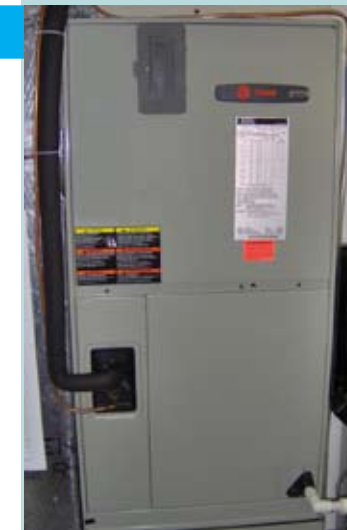
A 6-ton AC package unit used to sit on top of the roof and needed to be lifted off with a crane (far left). It was replaced by an 18-SEER, 3-ton Trane unit with a condensing unit that sits in the side yard and an air handler that fits into the hall closet (near left).
