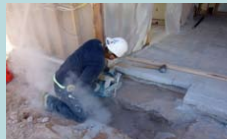
To install the holddowns for the Simpson StrongWalls, the slab edge had to be cut away (right) and reformed with an array of anchors.
