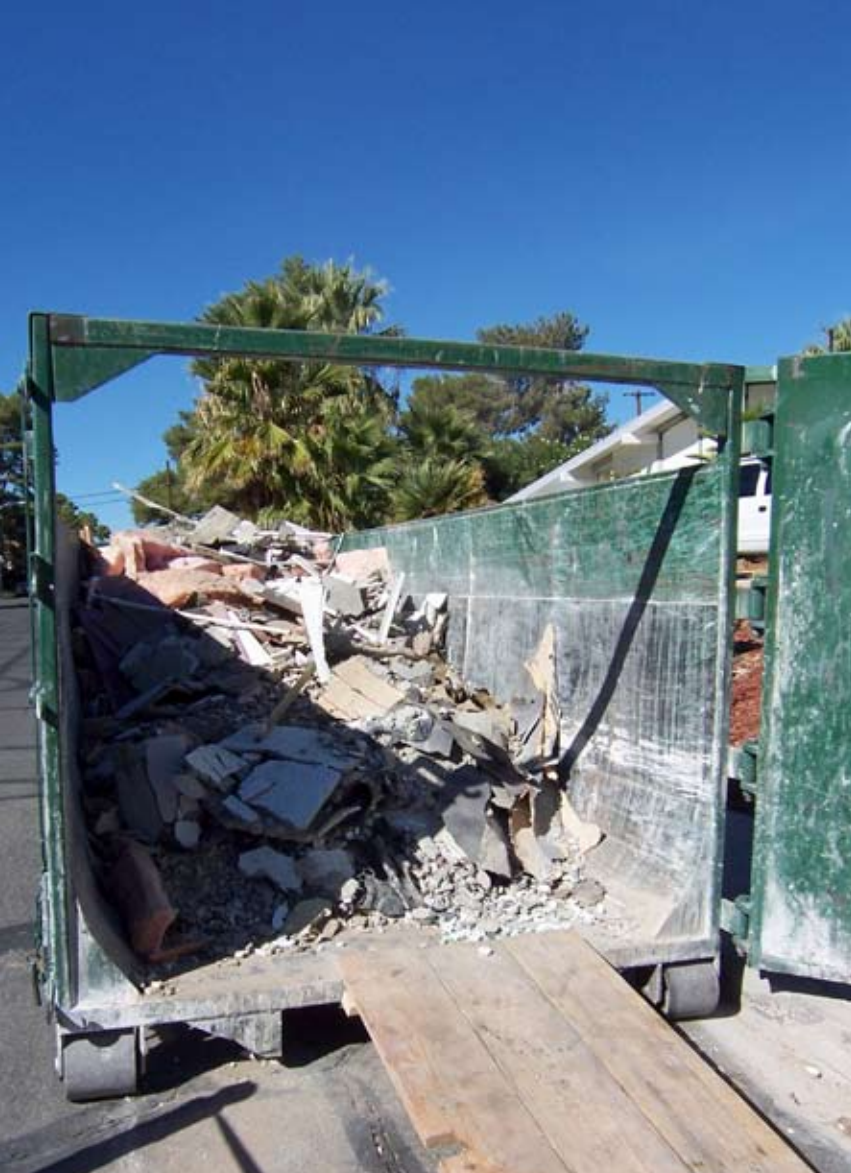
Evergreen Recycling collected site debris in unsorted dumpsters (left). By eliminating the sorting on site, no time was lost by the demolition crew.
