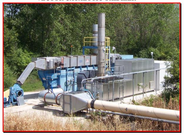
A chemical processing facility recently installed a VECTOR Catalytic Oxidizer to replace a competitors Regenerative Thermal Oxidizer. The RTO was installed 5 years earlier and could not provide the reliability demanded by the client. The problem stemmed from a basic *mis-application* of the technology. As is very common, many air pollution control equipment manufactures have abandoned recuperative technology in favor of focusing on regenerative technology.
