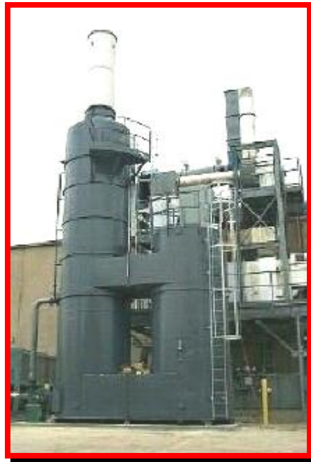
Photo is a QUADRANT SR-15,000 Silicone Series Thermal (recuperative) Oxidizer designed, manufactured and installed by Catalytic Products International, Inc.
