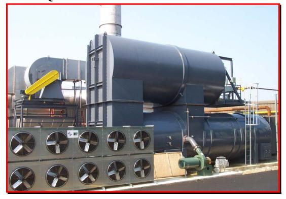
A synthetic leather manufacturer worked with Catalytic Products International, Inc. to design a unique Thermal (recuperative) Oxidizer. A recuperative thermal oxidizer was chosen because of high solvent LEL (+25%) exhausted from the process and a desire to integrate a hot oil recovery system to work with the oil heated production coating/curing line.
