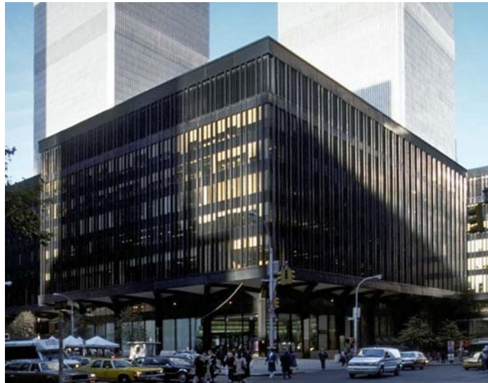
Figure 1. Exterior View of WTC 5.
