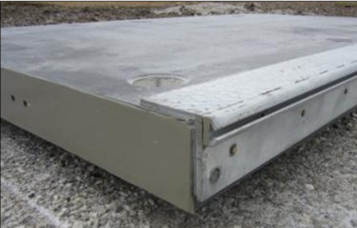
Panels at span ends have galvanized plate for impact resistance and expansion joint seals
