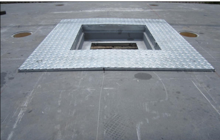
Manhole in deck for access to capstan under the swing span
