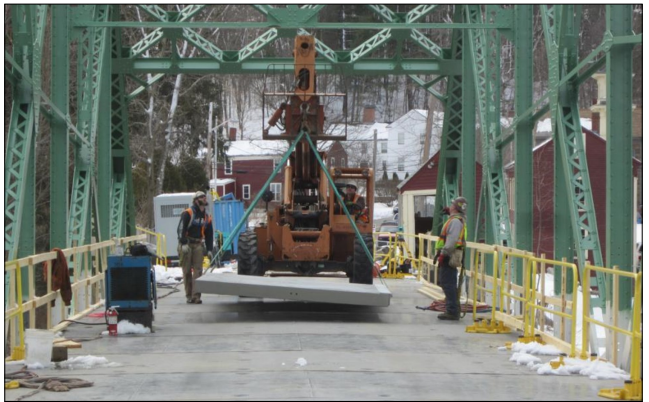
Deck Panel Installation using Light Duty Equipment
