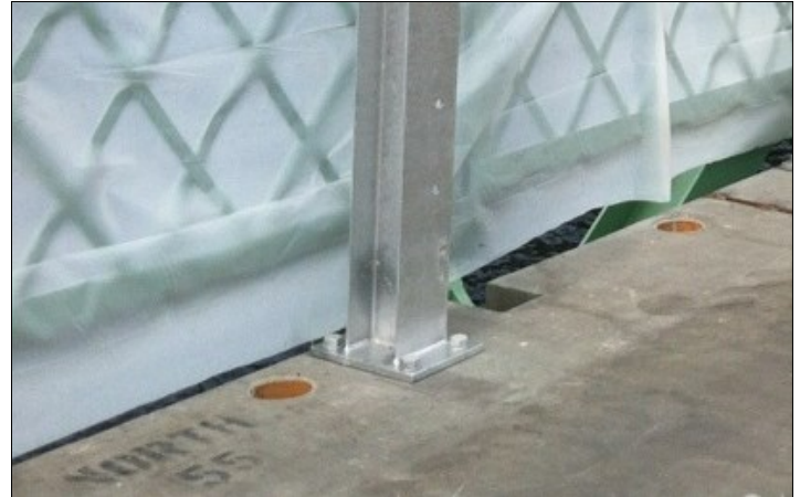
Guard rail attached to deck with internal steel reinforcement to react crash loads
