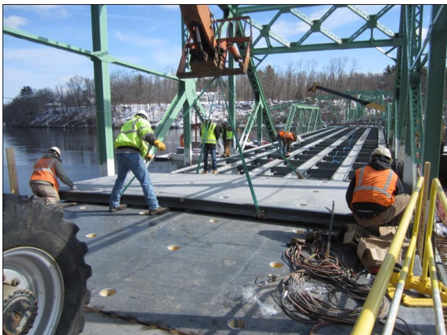
Deck Supported by Six Girders
