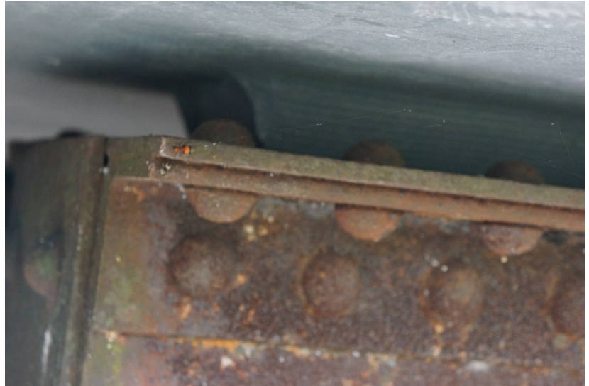
Molded spacer allows FRP deck to rest securely between raised rivets.
