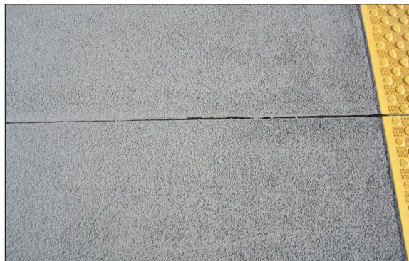
Panel to Panel Joint
