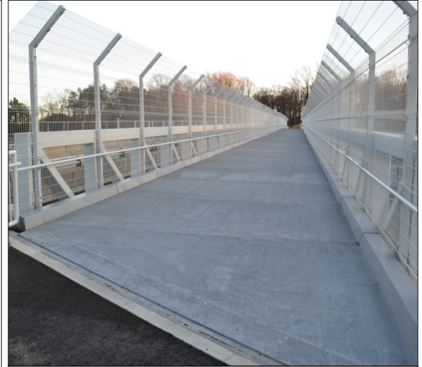
FRP Deck Performing Well
