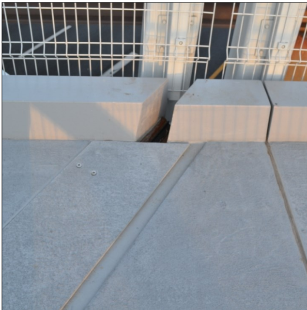
Expansion Joint Between Truss Spans and Panel-to-Panel Joints
