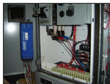
Figure 3: In addition to being rugged and reliable for use by non-expert operators, the ELITEpro SP instruments are compact enough to fit inside most electrical panels.
