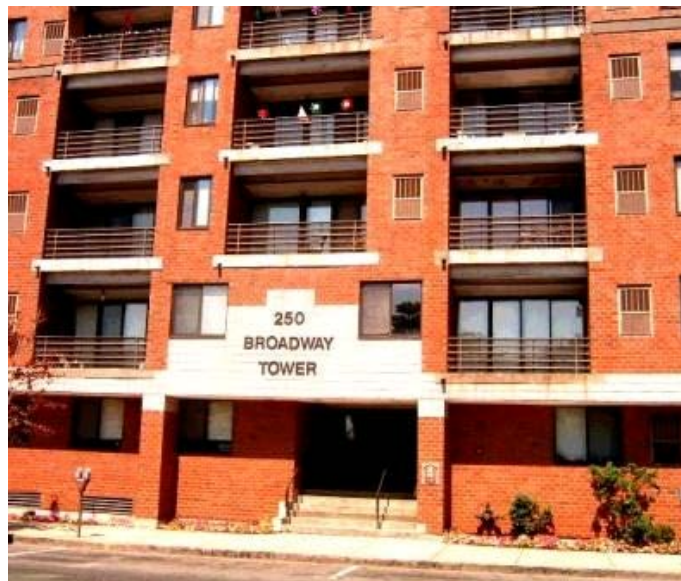
Figure 2. 250 Broadway Tower, Revere, Massachusetts
