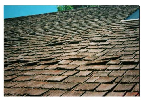
The main leak you are experiencing is a result of loose, missing and broken shingles in this area shown to the left. At this point in the life of your roof, 26 years old, we recommend a complete re-roof. You will not have to worry about this problem happening again for the life of the new roof. If you choose Lamarite composite slate shingles, the expected roof life will be 50 years!
